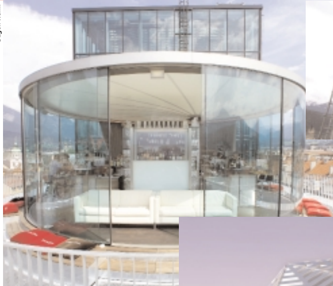
Above: Café Lichtblick, Innsbruck, Austria (2005). Walls of curved structural laminated glass give great, uninterrupted views of the surrounding Austrian Alps.
